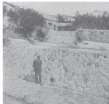
写真-10 愛知県瀬戸地方の練石積砂防堰堤(Hofmann, 1936より) Photo 10 Masonry check dams in Seto, Aichi pref., Japan (From Hofmann, 1936)
