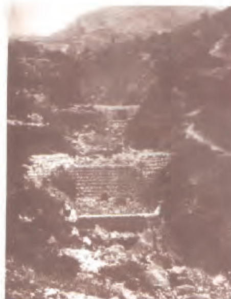
写真-3 ズヴィロニャック溪の砂防堰堤 (Martinović, 2015より) Photo 3 Check dams at Zvtronjak torrent (From Martinović, 2015)
