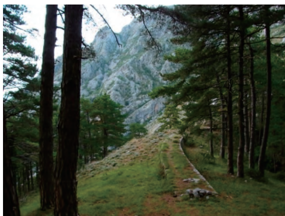
堰堤左岸の導流堤
