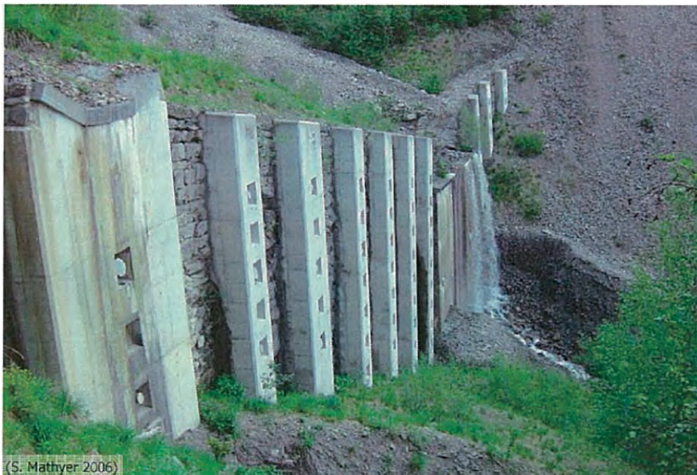
Lambach IVa Check Dam 12)
