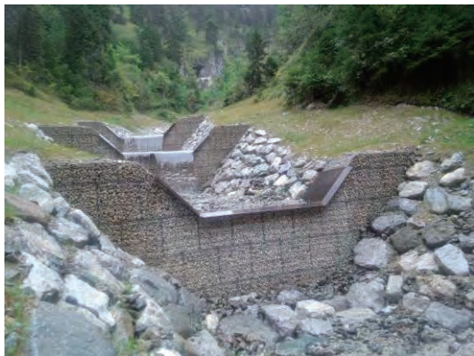
鋼製枠の砂防堰堤
