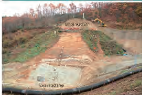
Fig. 2 View of field loading test site, 17 Nov 2000. The soil embankment reached 4.6 m deep
