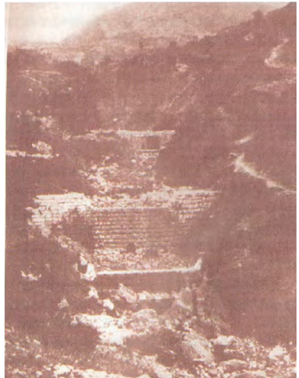
写真-3 ズヴィロニャック溪の砂防堰堤 (Martinović, 2015 より) Photo 3 Check dams at Zvironjak torrent (From Martinović, 2015)
