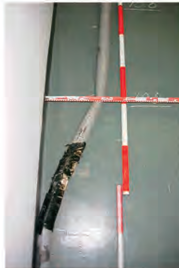
Fig. 9 Bent inclinometer guide pipe retrieved from inside the exploration shaft
